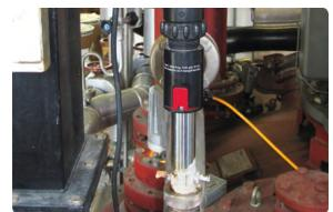
After more than 3 years of operation the Forbes Marshall pH sensor and RetractoFit are still in good shape and require only minimum maintenance.
