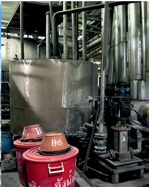
Condensate tank overflowing
