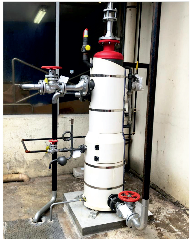
FlashJet™ Pump (FJP) enabling recovery of flash steam and condensate
