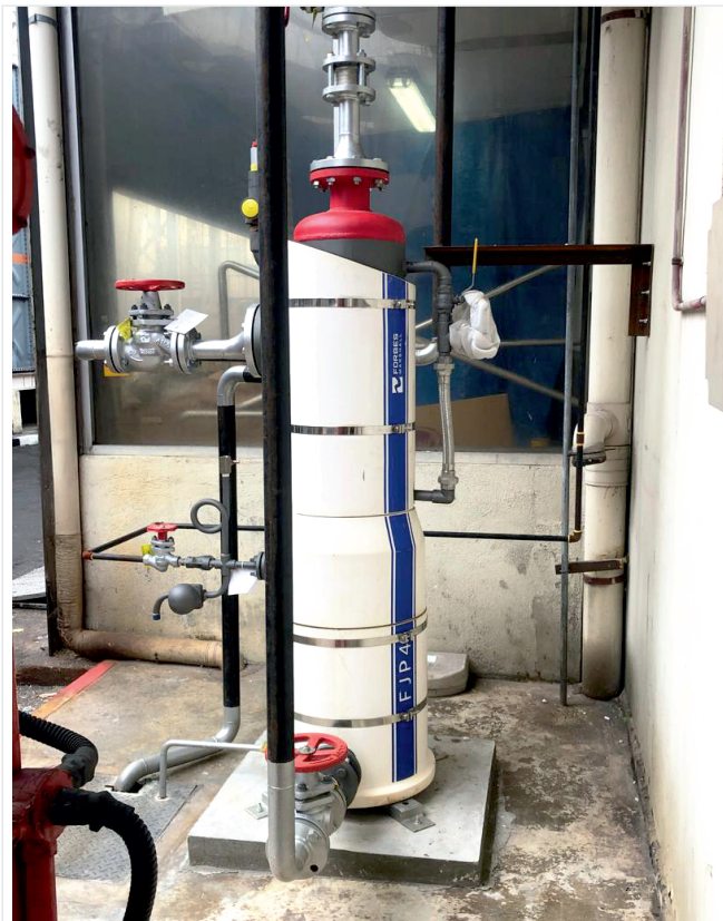
FlashJet™ Pump (FJP) enabling recovery of flash steam and condensate
