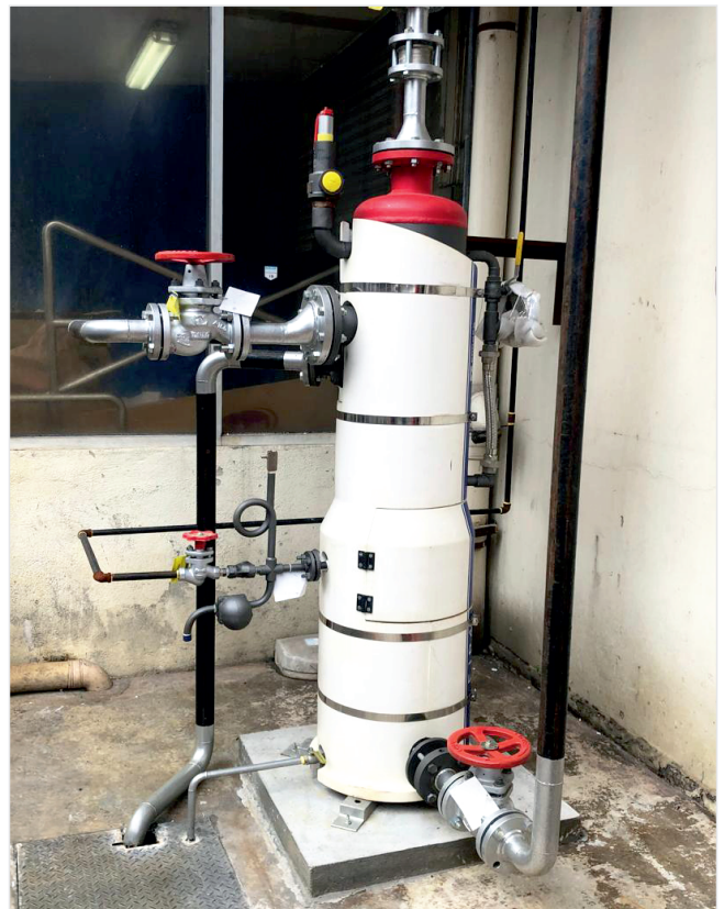
FlashJet™ Pump (FJP) enabling recovery of flash steam and condensate
