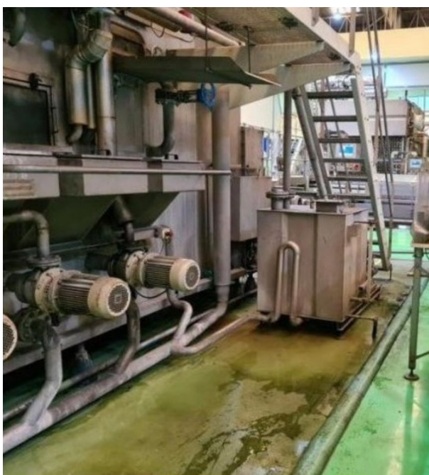
Condensate recovery by electric pump
