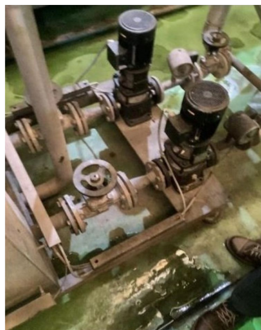
Condensate recovery by electric pump
