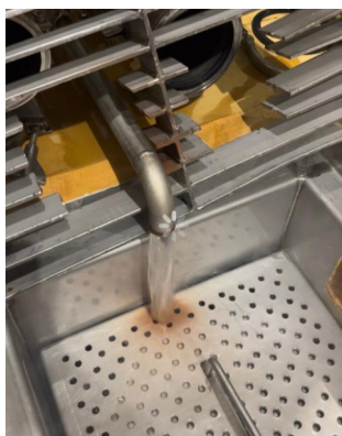
Condensate being drained locally by opening trap bypass valve
