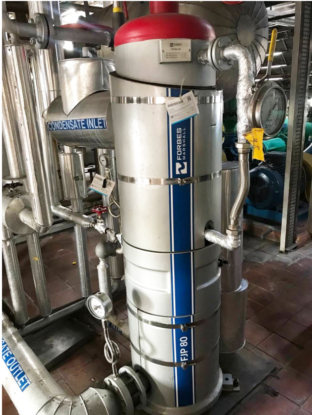
FlashJet Pump™ installation for condensate and flash steam recovery
