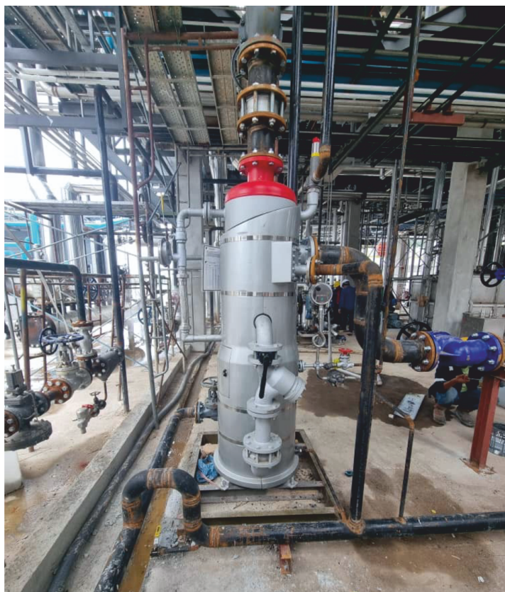
Forbes Marshall FlashJet™ Pump installation for condensate and flash steam recovery
