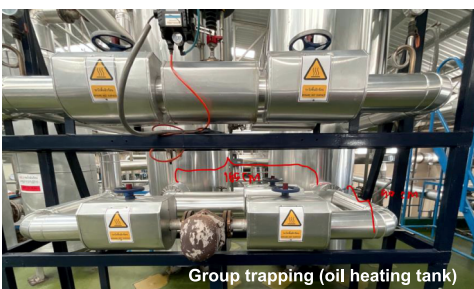
Improper sizing of steam header
