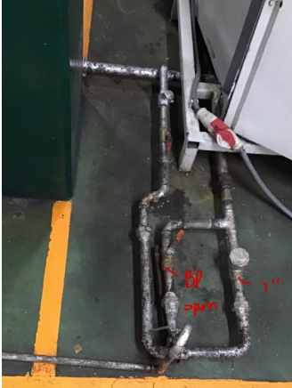
Wrong trap selection and bypass opening
