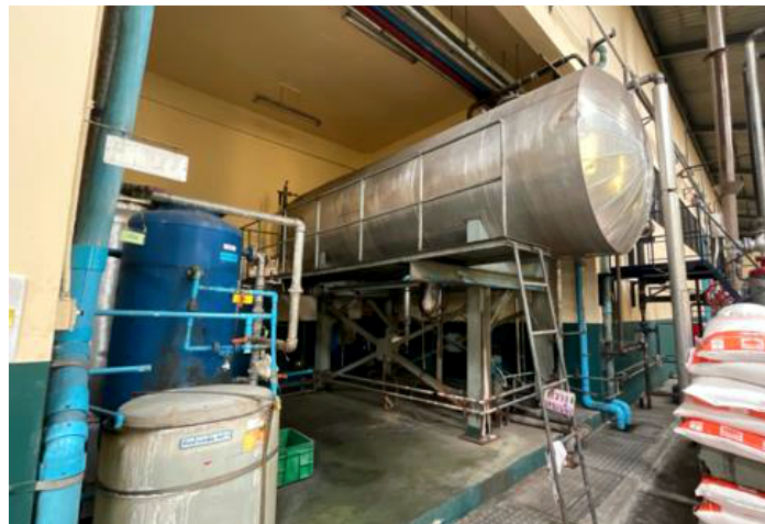
Condensate tank with electrical pump
