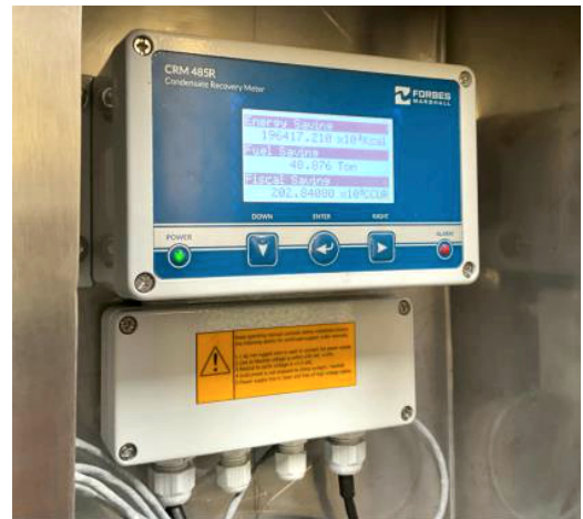
Condensate Recovery Meter (CRM) installed
