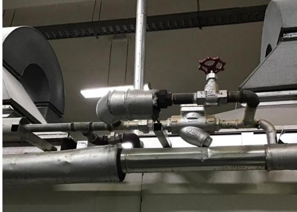
Wrong trap selection and group trapping
