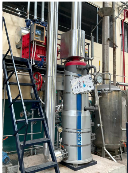
Condensate Recovery Meter (CRM) installed
