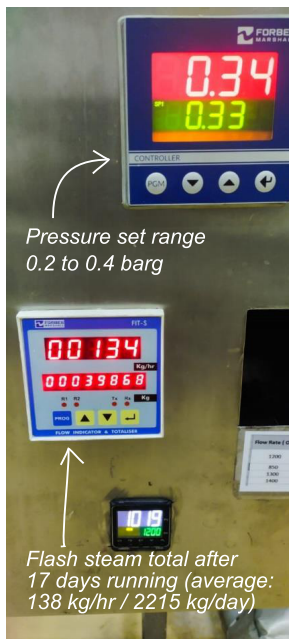
Pressure control system for Steamer, flash steam meter, and steamer meter
