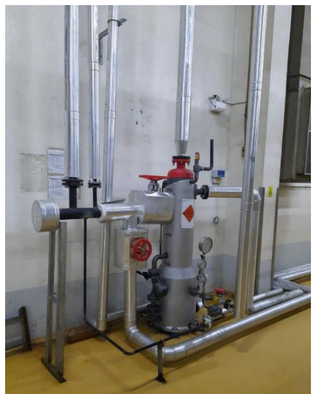
FlashJet™ Pump Installation
