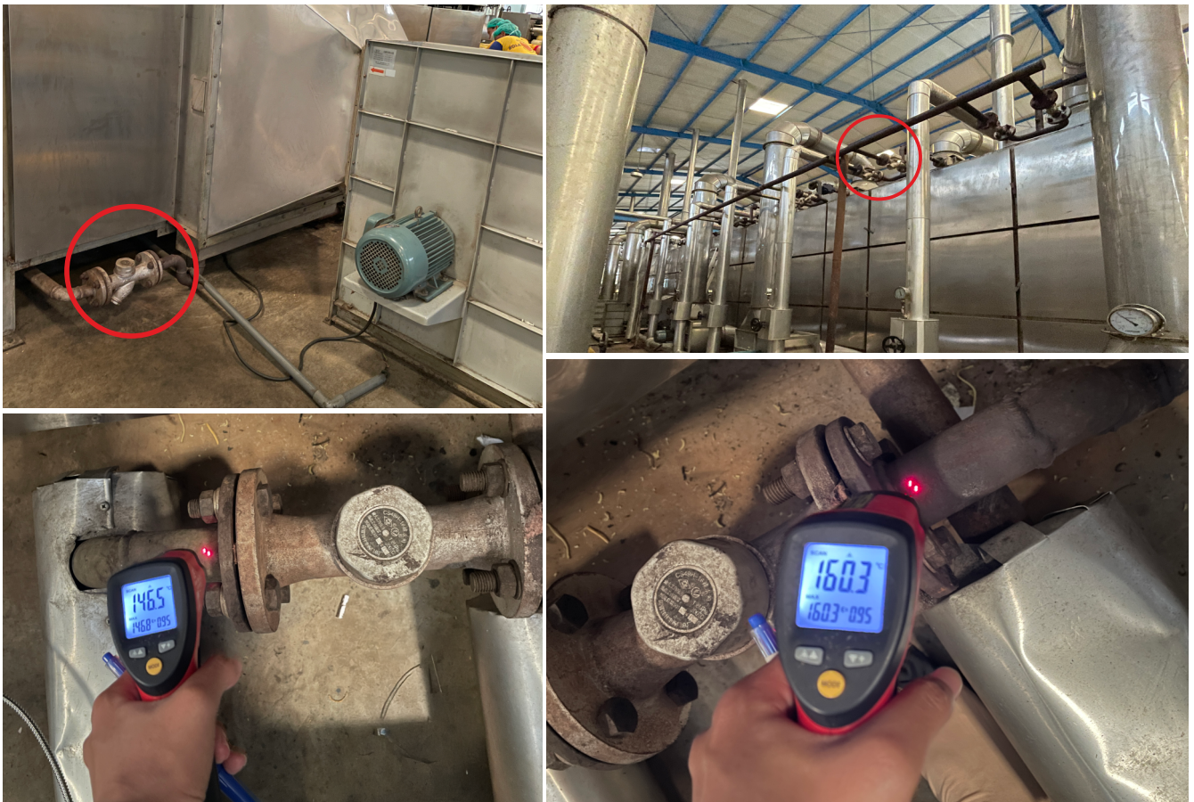
Dryer line 2 trap uptime at 0% due to incorrect selection of process traps
